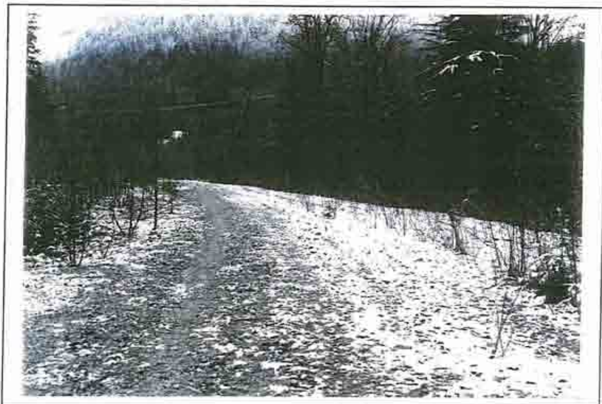
Photo 11 - Cascade Creek Dyke looking upstream near XS-5.
