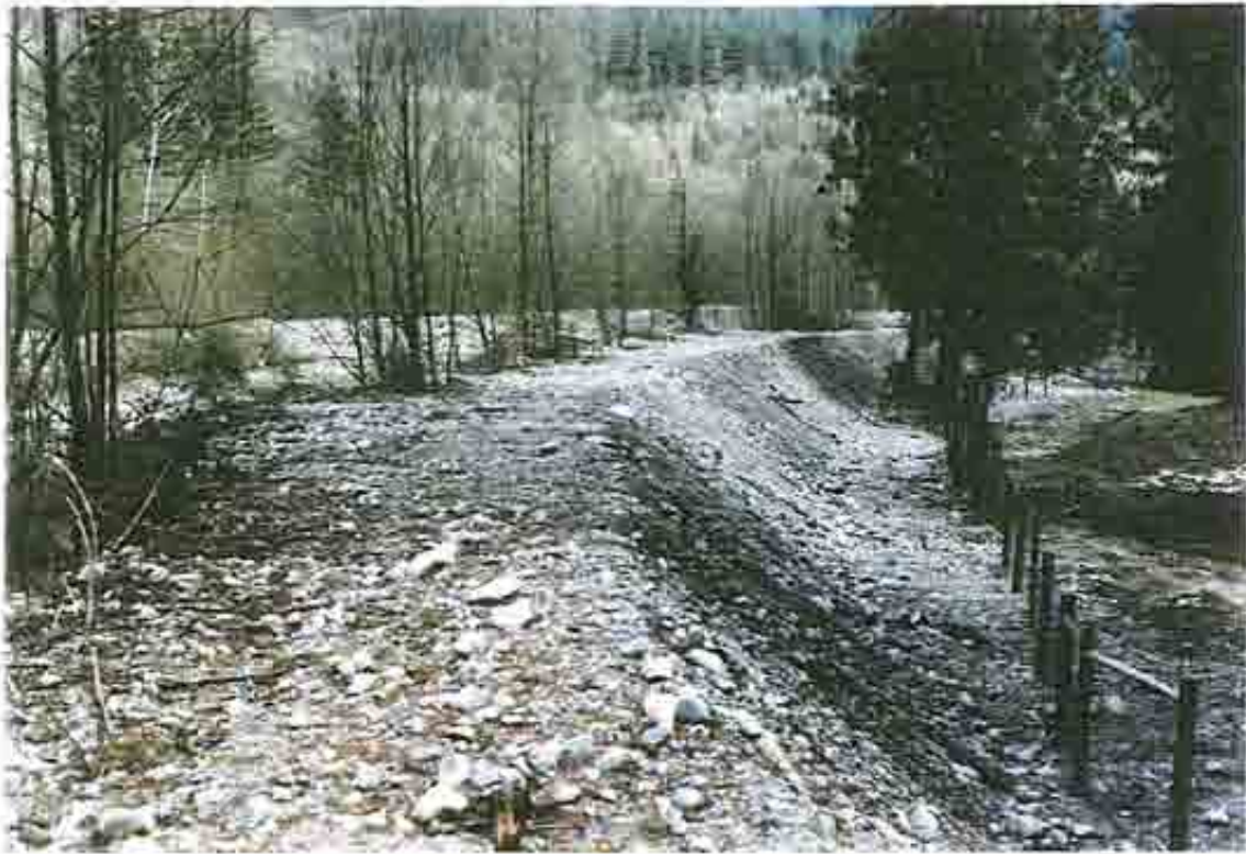
Photo 16 - Left Carratt Creek Berm looking upstream between XS-15 and XS-16.
