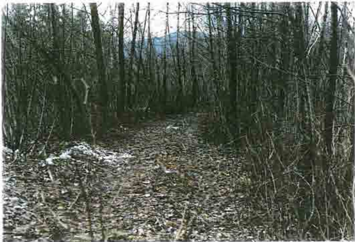
Photo 17 - Right Carratt Creek Berm looking downstream near XS-15.
